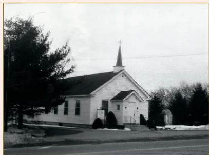
Figure 2 St. Mary of the Hills Chapel
